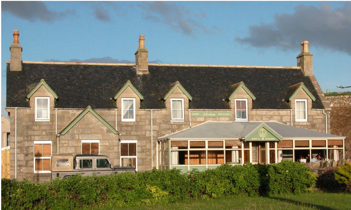
IMAGE 10 RENOVATED AND UPGRADED FORMER PARKHILL HOTEL MACKAYS ROOMS
