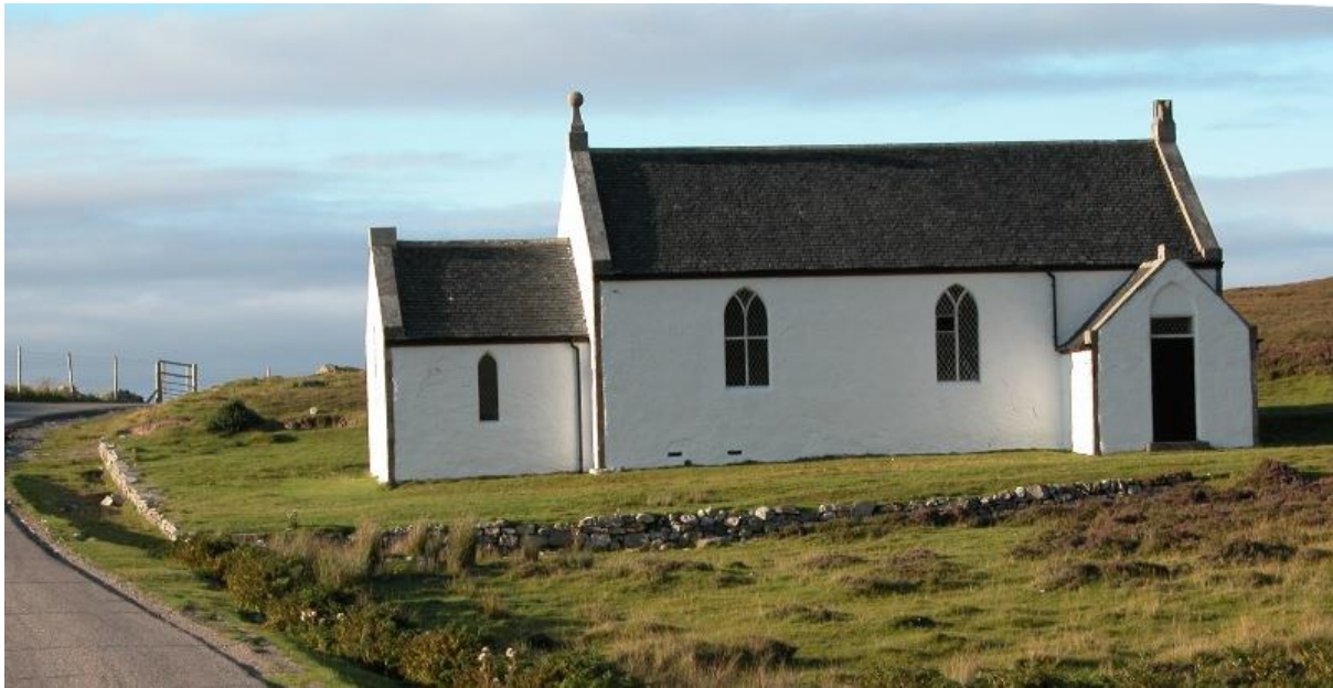
IMAGE 317 ERIBOLL CHURCH ON THE EASTERN SIDE OF THE LOCH
