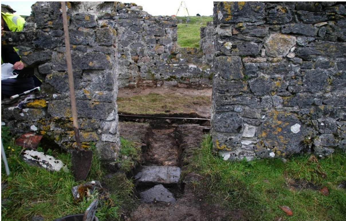
IMAGE 235 CROISPOL SCHOOLHOUSE TRENCH WAS OPENED TO GIVE A PEEK AT THE DOORWAY
